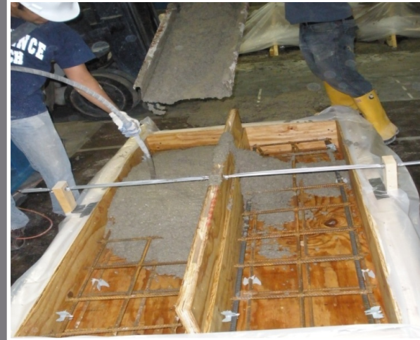
Concreting of Specimens
