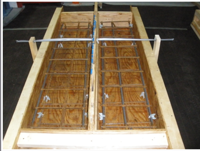
Reinforcement Cage & Form Work
