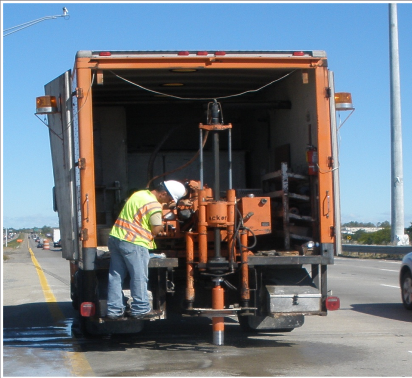
Coring full depth of the deck
